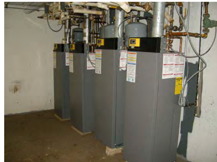
The combination heating and domestic hot water boilers
